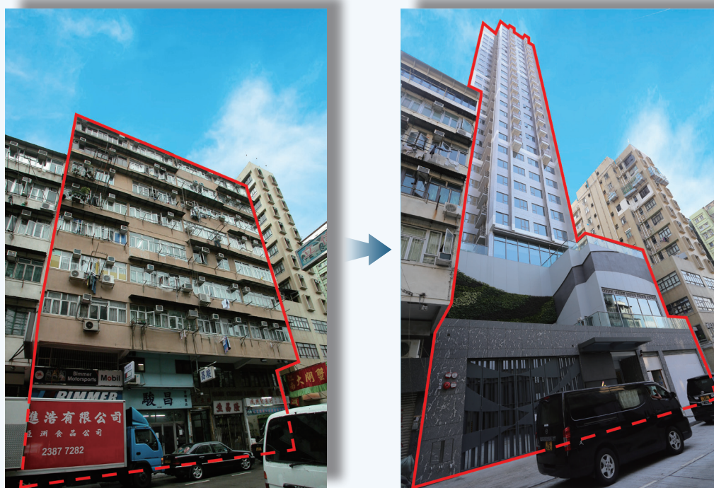
229A-G Hai Tan Street Development-Led Redevelopment Project (DL-1: SSP) – before and after redevelopment
