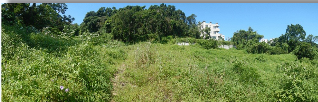
Excavation and Filling of Land Ceased and Land Reinstated after Enforcement Action
