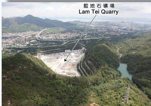
Lam Tei Quarry and the Adjoining Areas
