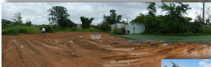
Hard Paving Removed
