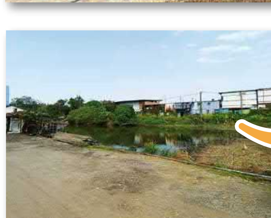
活化后的新田西主排水道 Revitalised San Tin Western Main Drainage Channel
