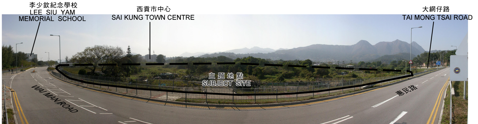
由東面拍攝 VIEWED FROM EAST
