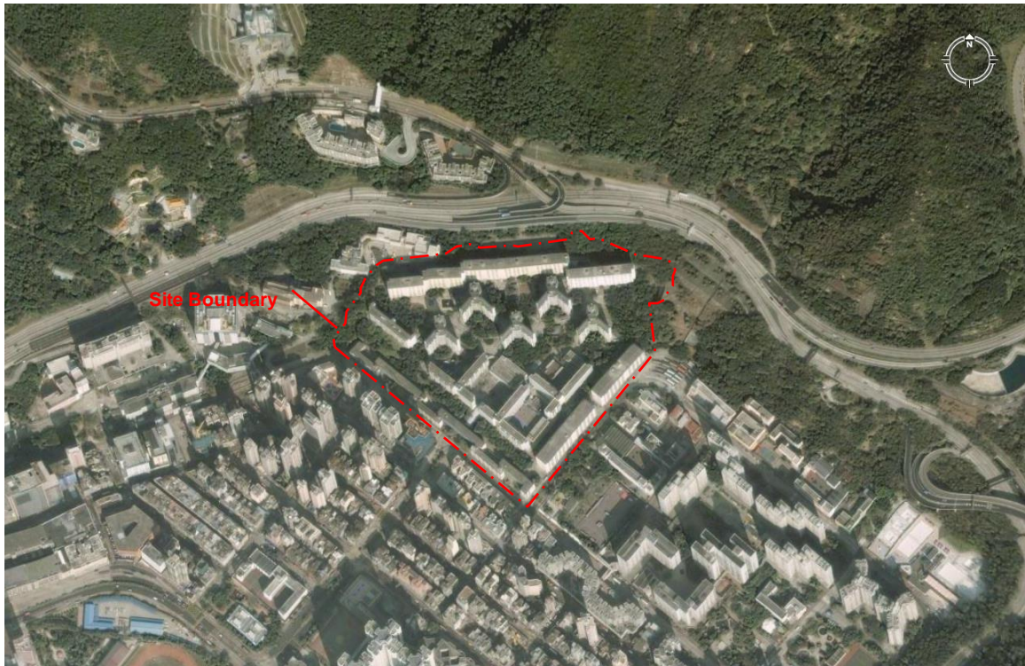
Figure 4 Existing site condition of So Uk Estate
