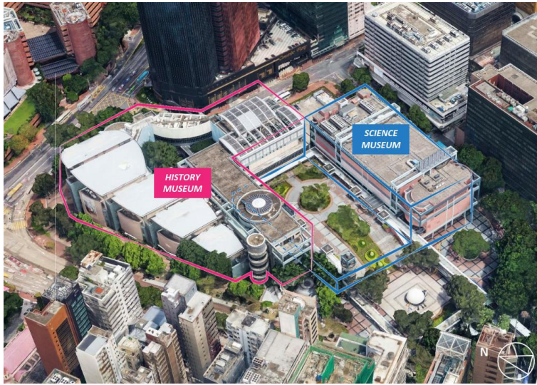
Figure 2 The Existing Buildings in the Subject Site
