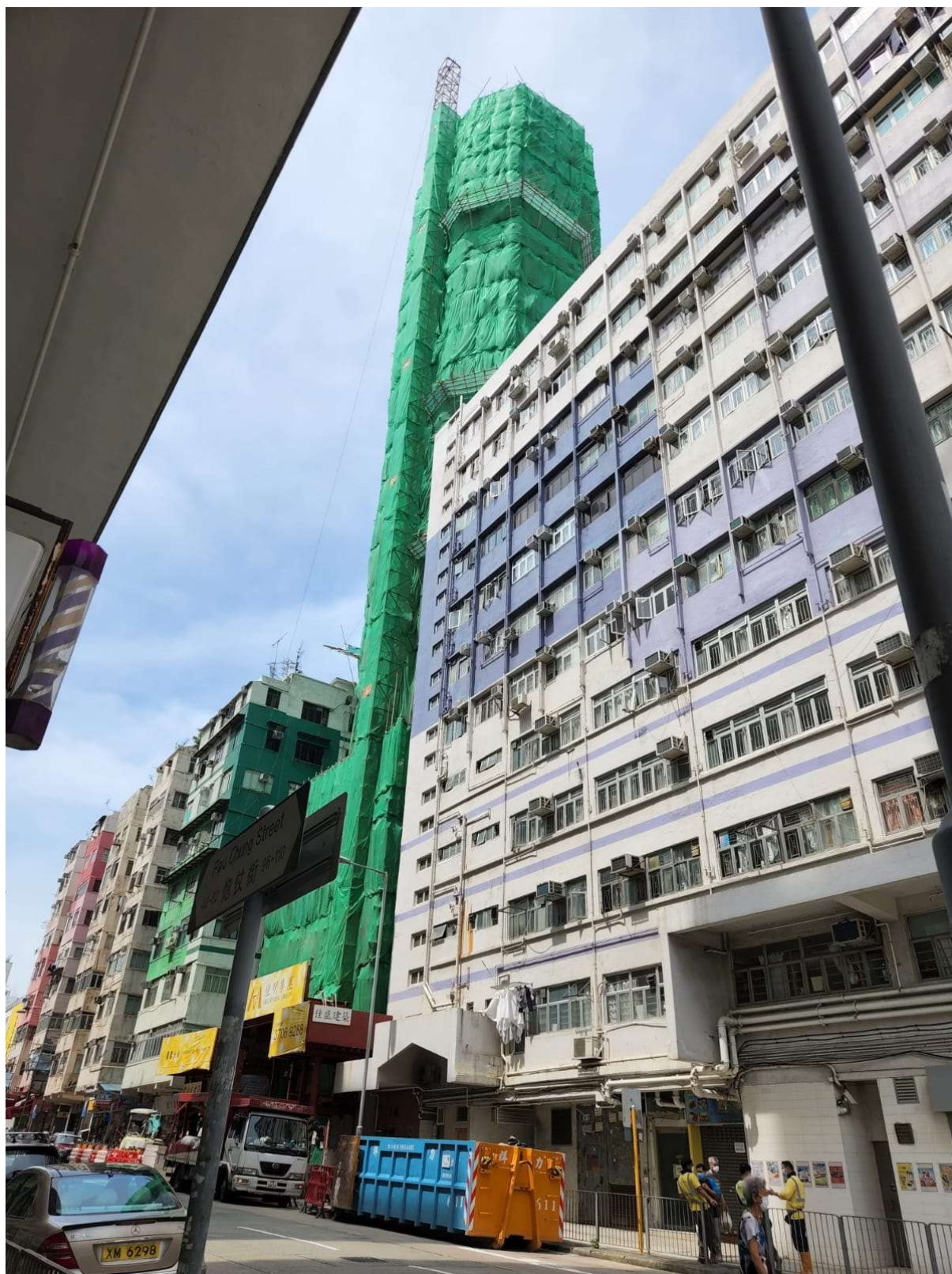
2. 41, 43 and 45 Pau Chung Street
