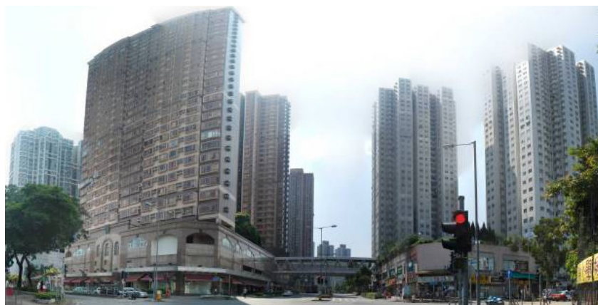
Figure 10: Ma On Shan Town Centre
