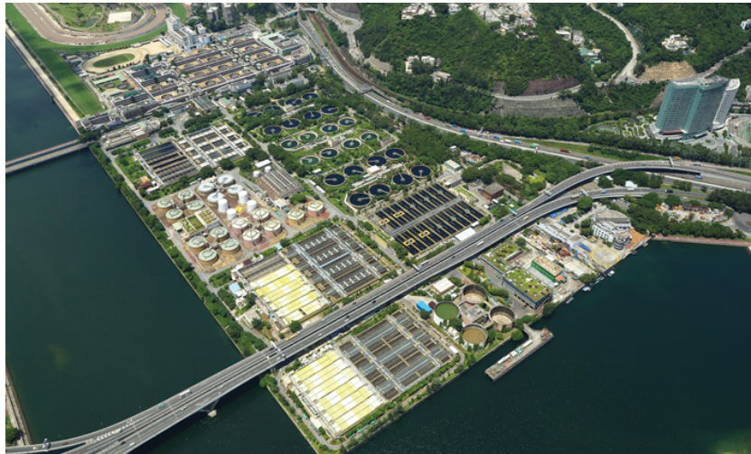
Figure 16: Existing Sha Tin Sewage Treatment Works
