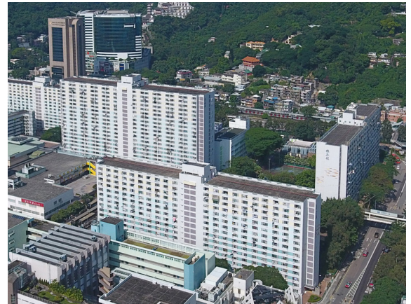
Figure 2: Lek Yuen Estate
