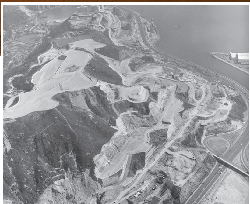
Figure 3: Excavation of fill materials from the nearby hill in Kwai Chung for reclamation
