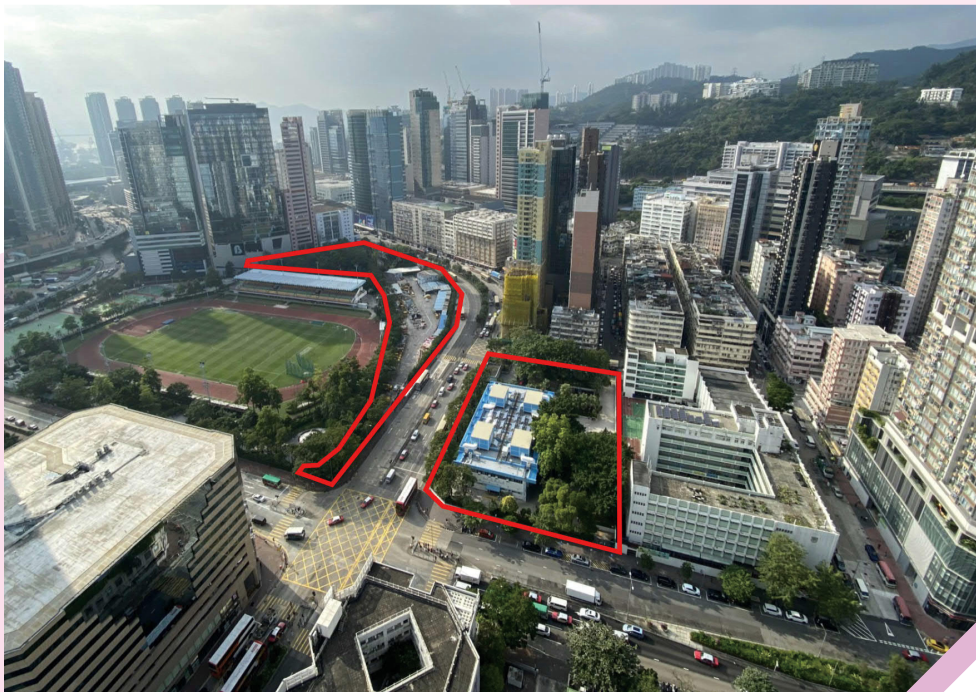
Cheung Wah Street/Cheung Sha Wan Road Development Scheme Site (SSP-018)
